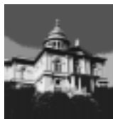
Cover: Placer County Courthouse Auburn, California
